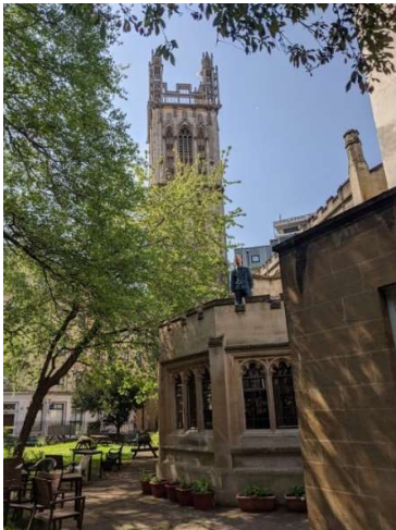
Dave checking for leaks on roof
